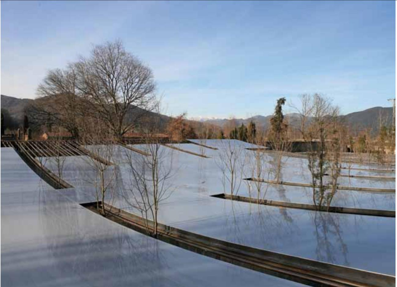
PROFITER D'UN GRAND ÉVÉNEMENT DANS UN ESPACE PROTÉGÉ PAR UNE COUVERTURE EN CLAIE DE ROSEAUX, TELLE FUT LA VISION DE L'ARCHITECTE POUR CRÉER CET ESPACE. IL EN RÉSULTE UNE COUVERTURE EN **ETFE** TRANSPARENTE ET LÉGÈRE, AVEC UNE STRUCTURE D'APPUI MÉTALLIQUE SPÉCIALE, LE TOUT DANS UN ENVIRONNEMENT SINGULIER.
